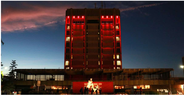
A new lighting system allows for Brock's Schmon Tower to glow in various colours at night.
