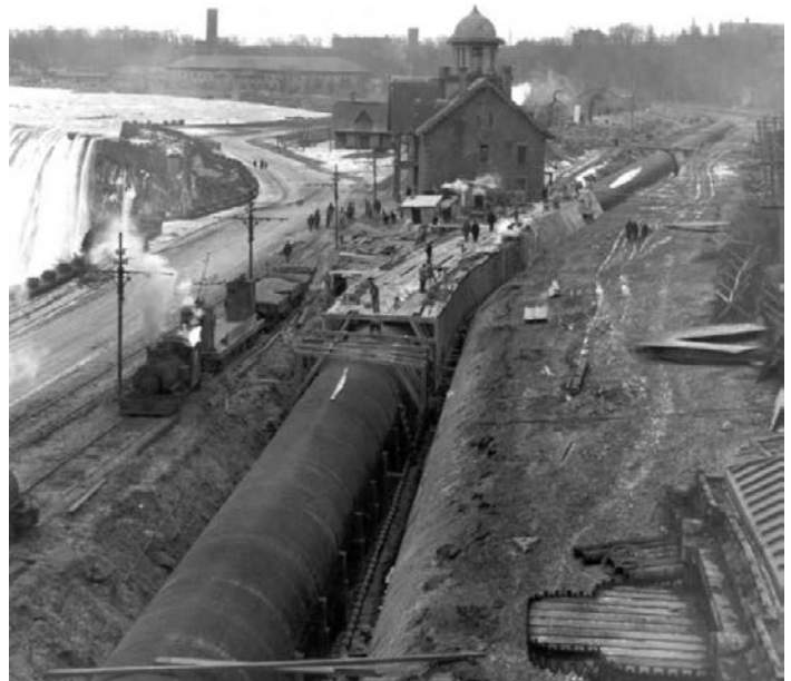
Laying power conduit along the parkway, c. 1905. Courtesy Niagara Railway Museum.
