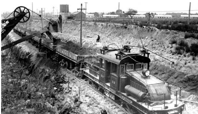
Electric locomotive c. 1918 during the construction of Sir Adam Beck G.S. #1. Courtesy Niagara Railway Museum.
