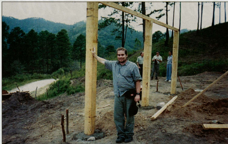
Brock grad Tom McLagan stands next to the frame of a house that was being built to help a needy family in Honduras.
