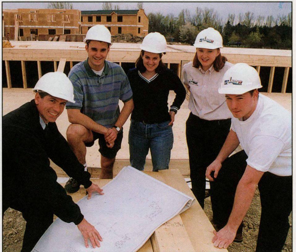
Jamie Fleming, Director of Residences, points to a blueprint of the addition to the Village Residence. With him at the construction site are students, from left, Mike Greenwood, Andrea Palko, Marie Hackett and Darren Fox.
