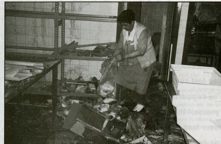
Sterilization Unit, Main Surgical Trauma Centre, Kosevo Hospital, Sarajevo. An artillery shell had hit twenty minutes earlier.
