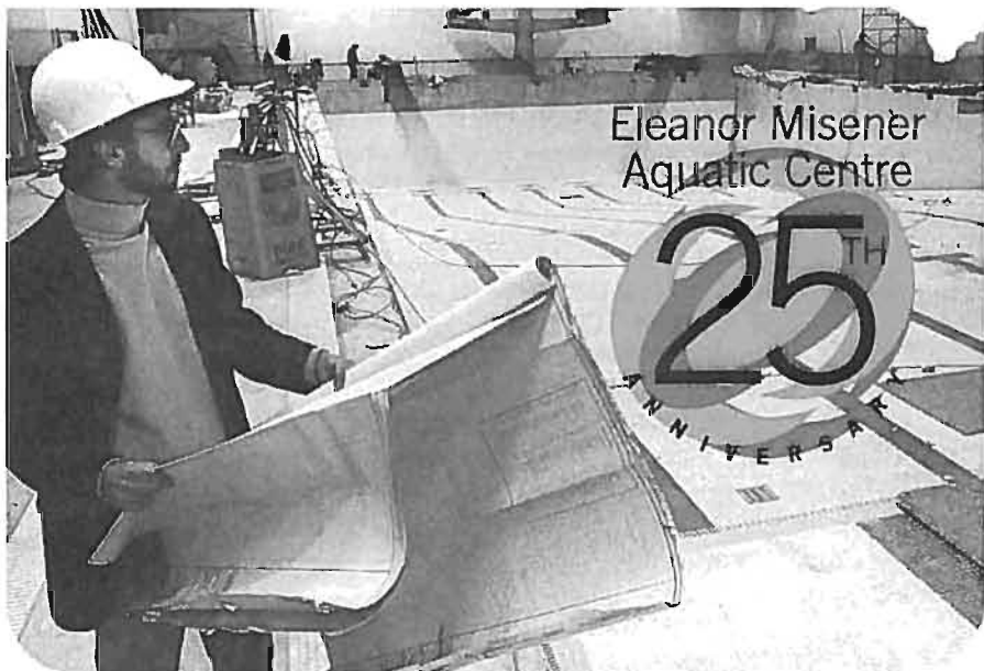
Herb DeBray, Manager of the Eleanor Misener Aquatic Centre, looks over the construction of the pool in 1980. DeBray still serves as Aquatics Manager, and is looking forward to celebrating the 25th anniversary of the centre during Brock Days.
