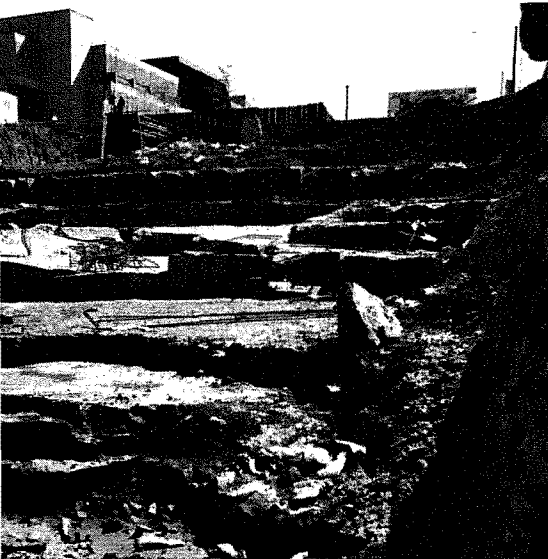
It may not look like a swimming pool yet, but construction is scheduled to be finished in late spring.
