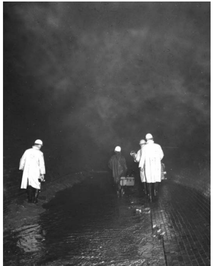
The Canadian Niagara Power Company generating station’s tailrace tunnel. Courtesy Brock University Archives and Special Collections.
