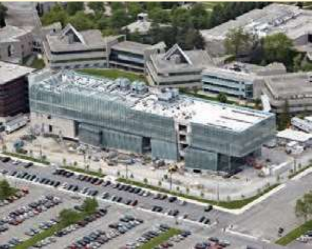
Work continues on the Cairns Family Health and Bioscience Research Complex.
